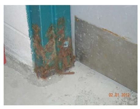
Corroded Door Frames Compromise Fire Rating
